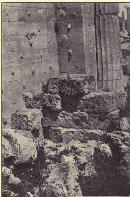
FIG. 20.—Anathyrosis from wall of Propylaea, Athens.
